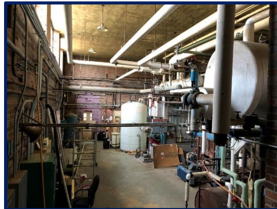
School Mechanical Room
